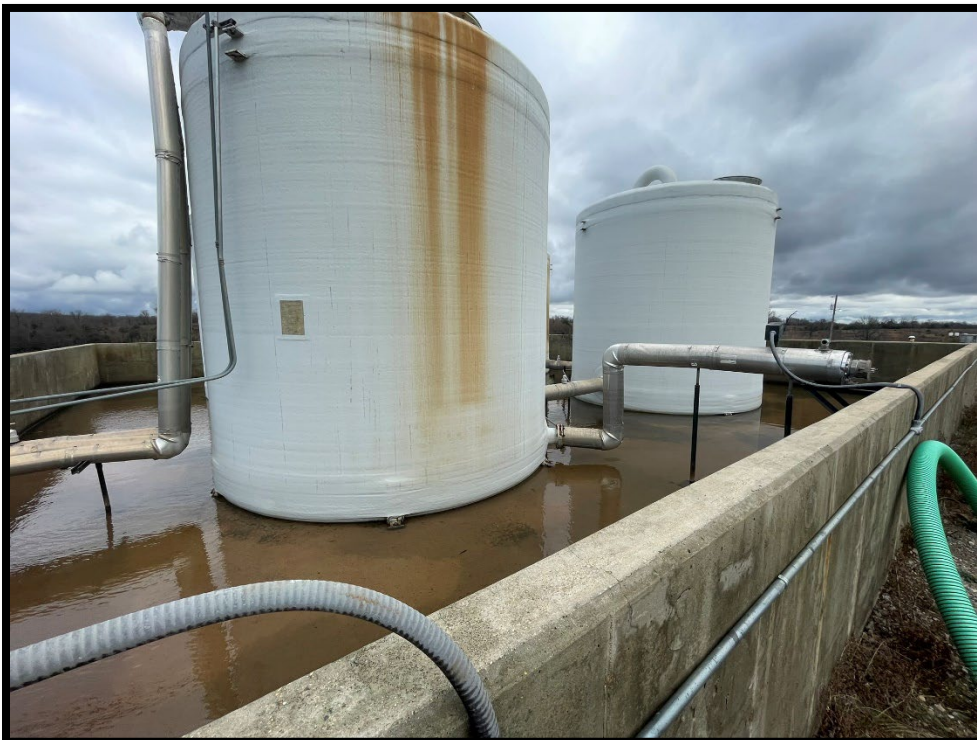
Photograph 2: View of stormwater in secondary containment at leachate tank battery.
