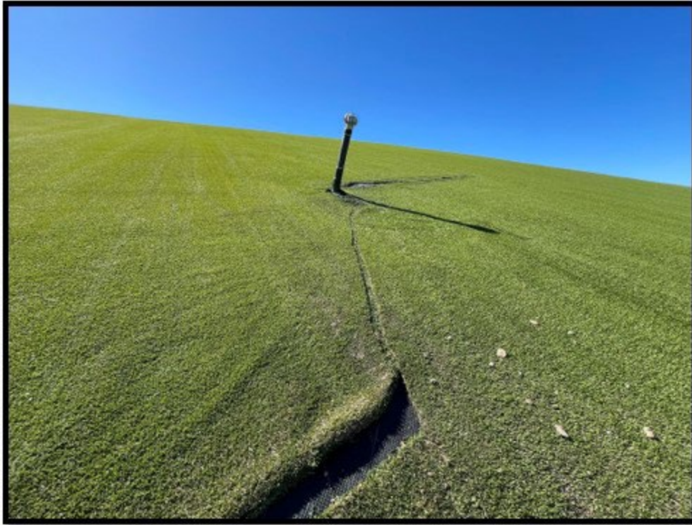
Photograph 5: View of damaged closure turf on the north side of Area 1-2.
