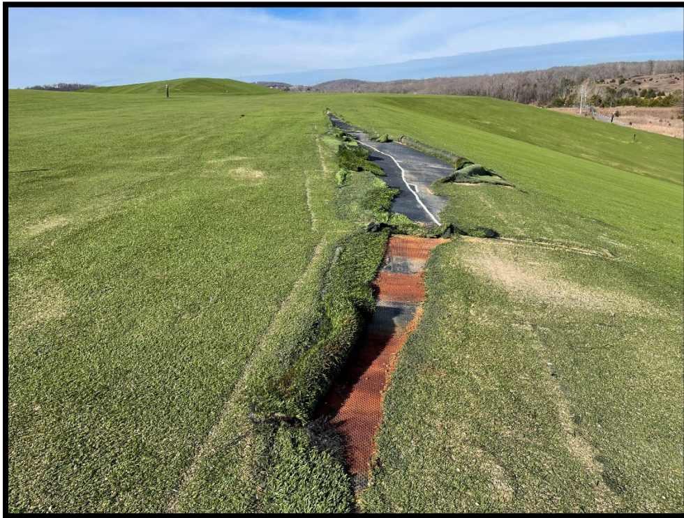
Photograph 6: View of damaged closure turf on east side of Area 1-3.
