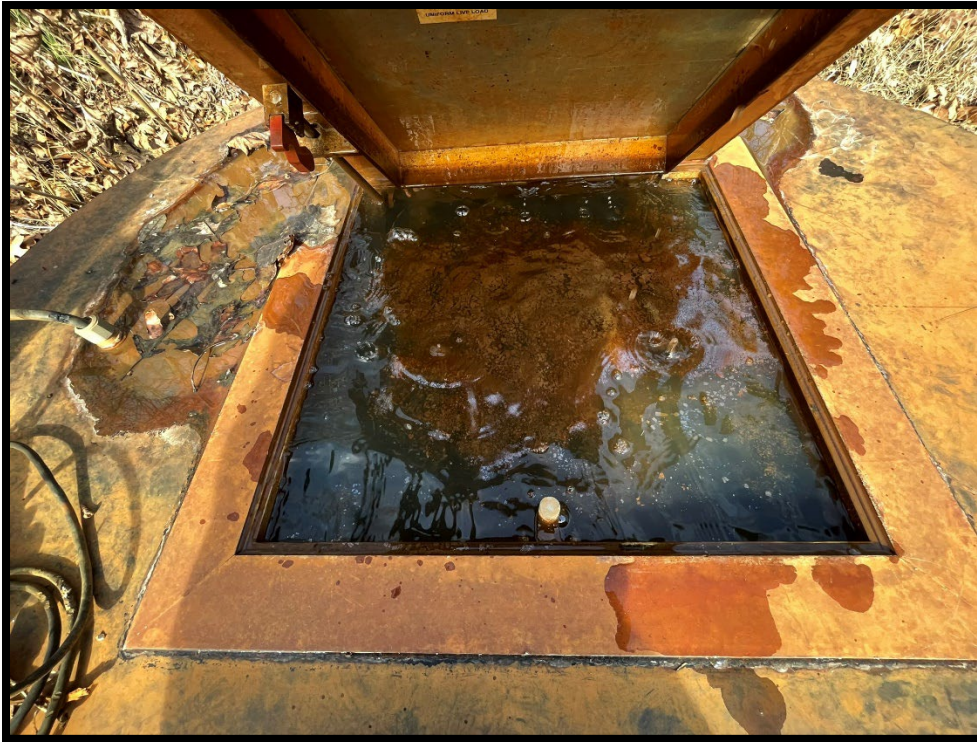
Photograph 1: View of VLCS-1 at capacity and overflowing.
