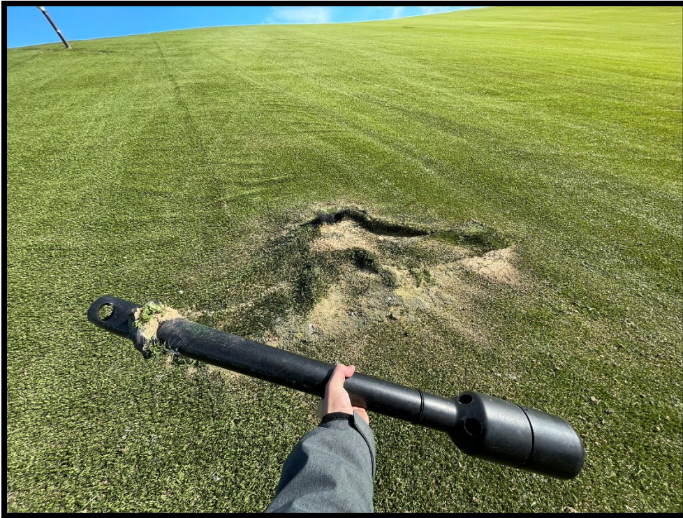
Photograph 3: View of first damaged pressure relief vent on west side of Area 1-2.
